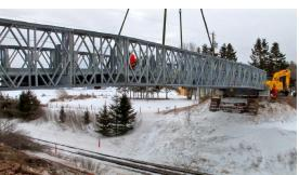
View this drone video showing the ROW rail crossing with cambered end sections to help with doublestack rail car clearance
