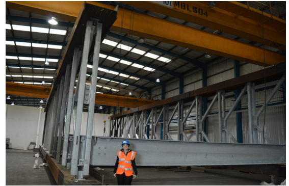
Section of an MTQ 100+ m bridge
