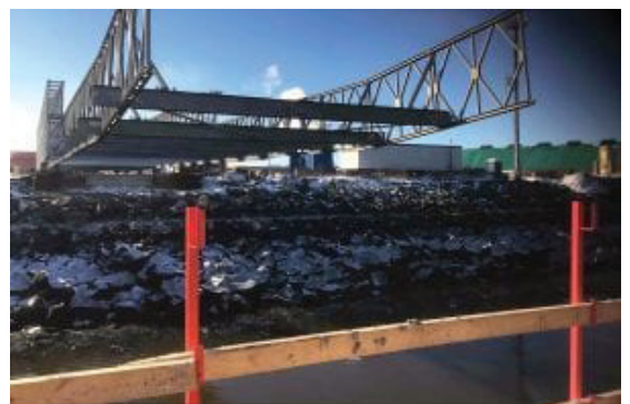
Nose module reaching prepared foundation on opposite side.
