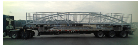
Each bridge delivered on a flatbed trailer and installed in one day
