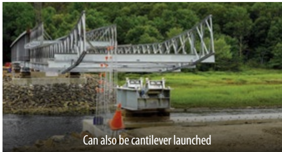
Pre-cambered side trusses
