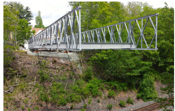
No heavy-lifting equipment: Algonquin Modular Panel Bridge cantilever launches over active rail line
