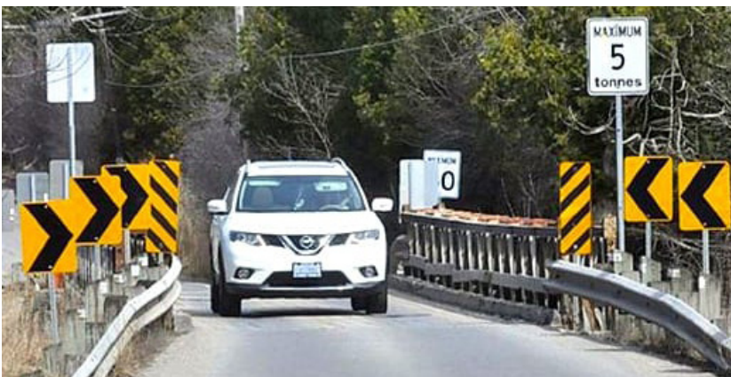
Replaced a 40-year-old "temporary" Bailey Bridge
