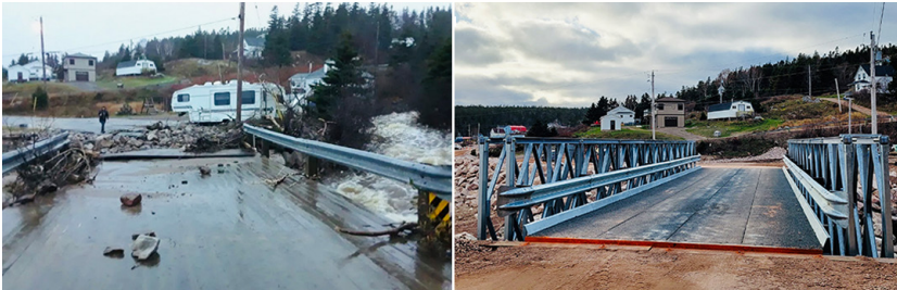
The original wooden bridge sustained substantial damage
