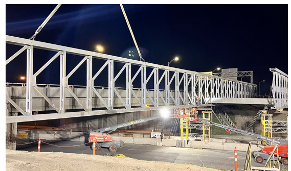
Night installation of Modular Bolted Truss Bridge at Boulevard Masson
