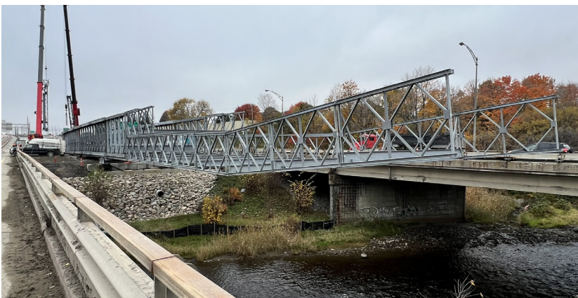
Cantilever launch of Modular Bolted Truss Bridge over Saint-Charles River
