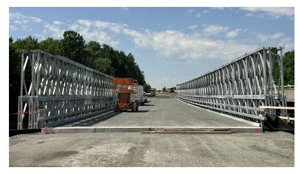
Our made-in-Canada R800 Modular Panel Bridge System is being used for a longer-term, 18-month rental detour bridge in support of a bridge rehab project on busy Autoroute 20 at Notre-Dame-du-Bon-Conseil, QC. The span reaches 70 m over the Rivière Nicolet Sud-Ouest.
