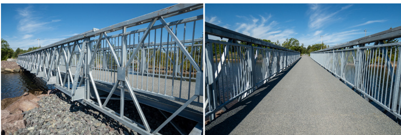
Vertical picket safety rails and anti-slip decking on R800 Modular Panel Bridge
