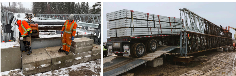
Left: Precast concrete blocking for adjustable approach ramps. Right: Example of an adjustable approach ramp used in our bridge testing.
